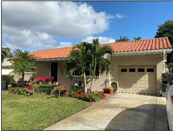
Figure 5: Noncontributing property at 2401 Andalusia Way NE
