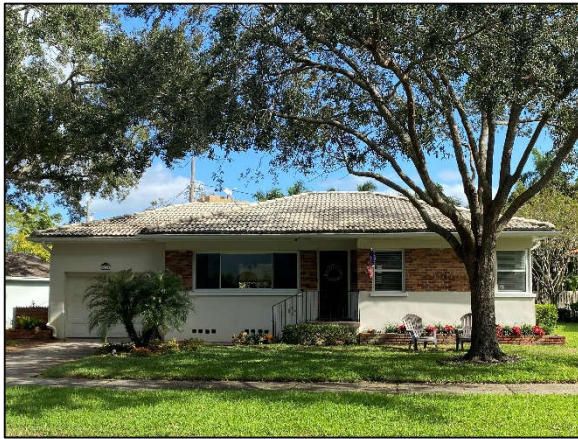
Figure 7: Noncontributing property at 2411 Andalusia Way NE
